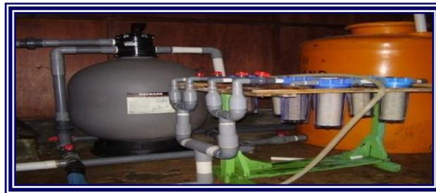
Gambar 15. Sanfilter Cartridge
