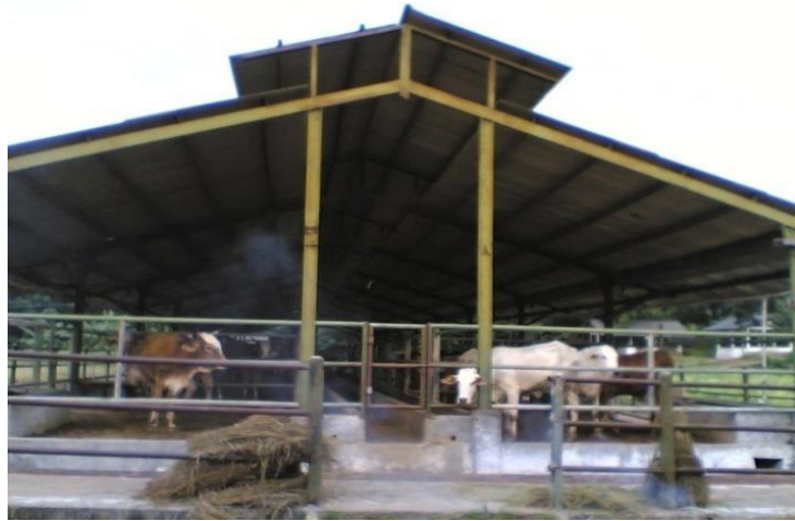
Gambar 2. Kandang Sapi atap model monitor
