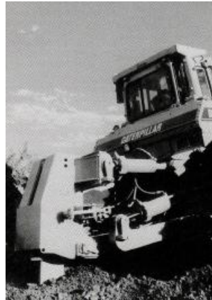
Gambar 6.3 Operasi dozer saat ripping
