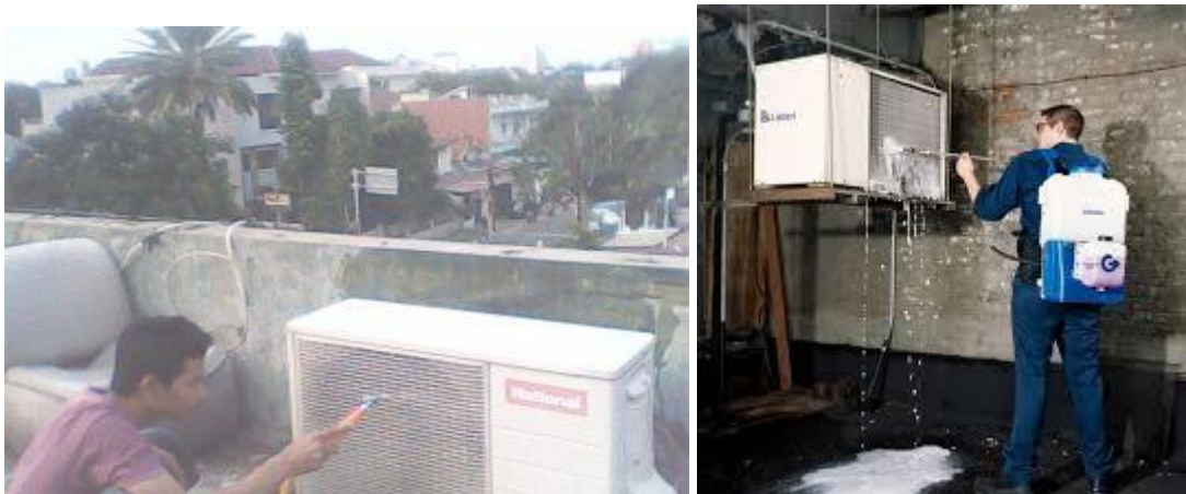
Gambar 3.19 Pembersihan Outdoor unit
