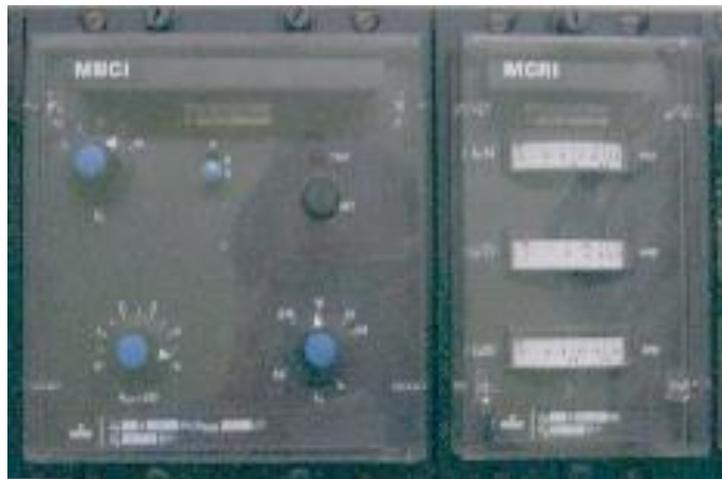
Gambar 3-19. Relay Differential Pilot Kabel.
