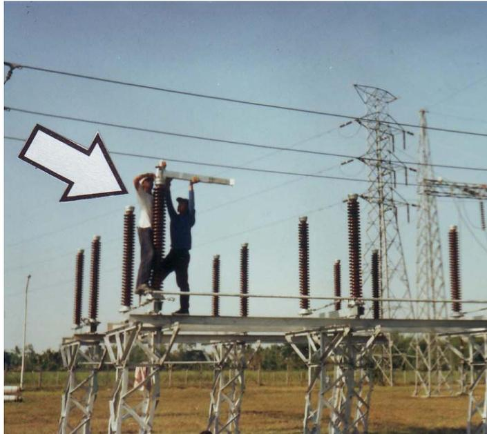
Gambar 3-4. *Disconnecting Switch (DS).*
