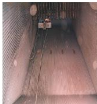
Gambar 3.4 Wall tube boiler
