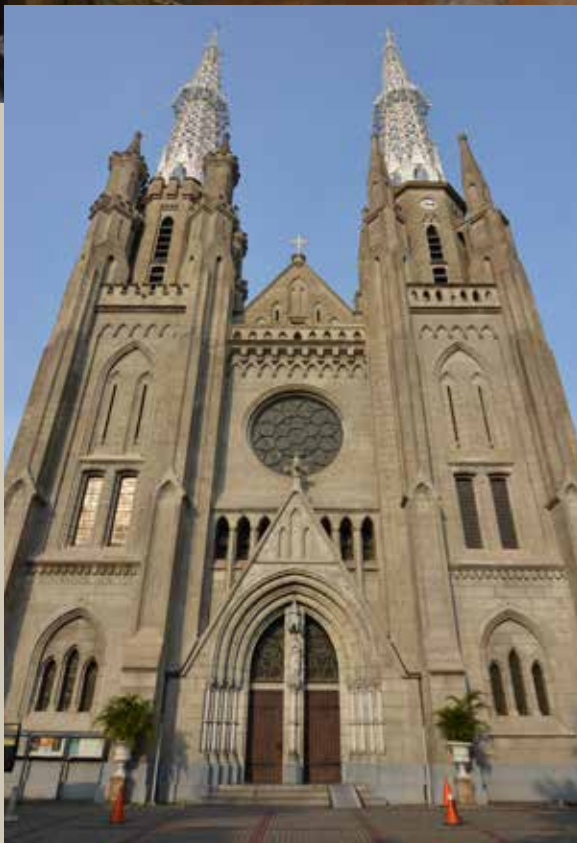
Bangunan Gereja Katedral The Cathedral Church Building
